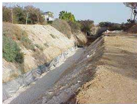
Figure 1: Open trench where tailored bacteria/carrier materials will be introduced for semi-passive treatment of drained pesticide-containing water.
